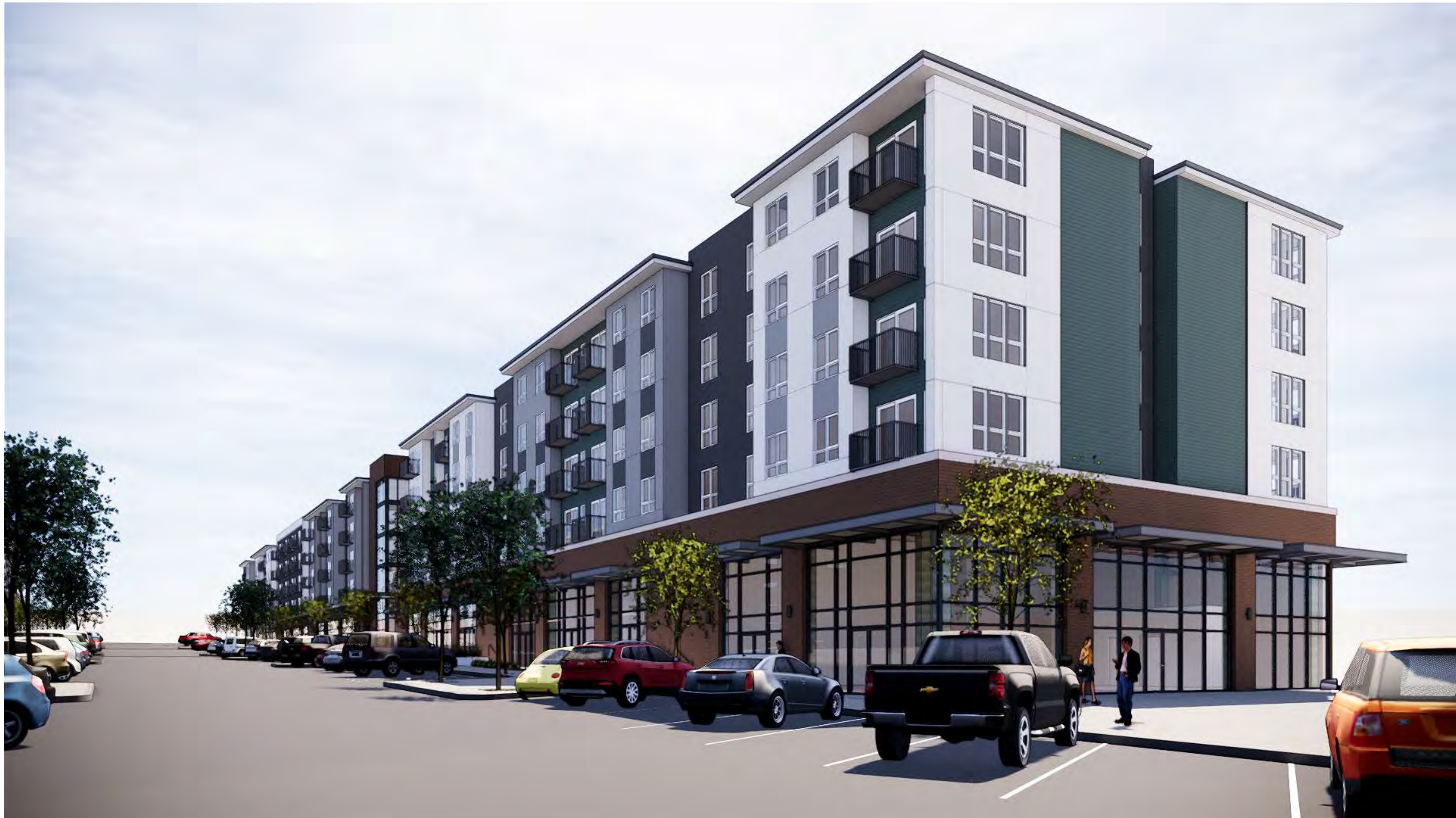
BUILDING E LOOKING SOUTH EAST
