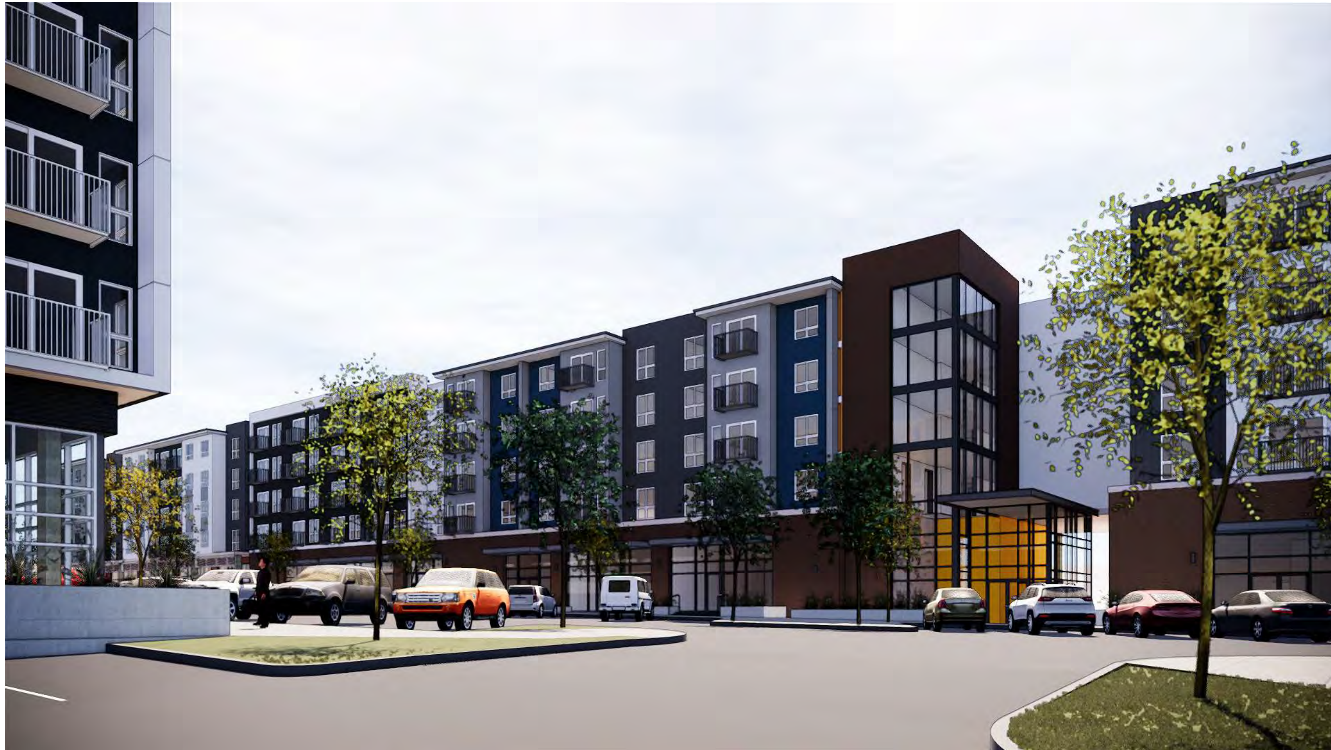
BUILDING E LOOKING SOUTH EAST
